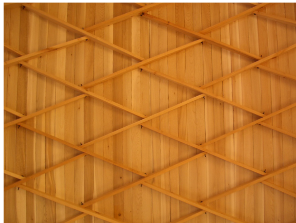
Figure 4: Characteristic diamond pattern of a lamella roof
