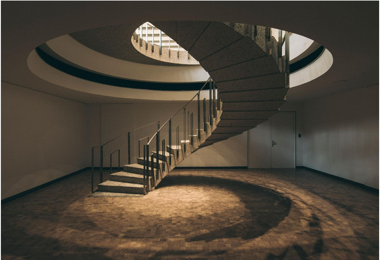
A spiralling concrete staircase conceived by Brodzki for the CBR HQ in Brussels
