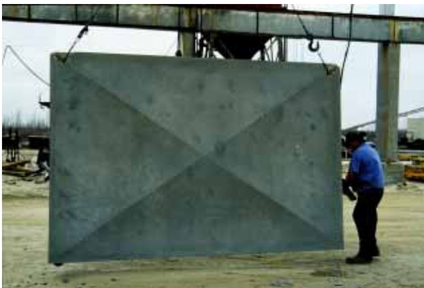
Figure 9. Lightweight compression vault panel cast from the inverted Figure 3 formwork shown in Figure 8 above. This panel varies in thickness from 38 mm (1.5 in.) to 127 mm (5 in.).
