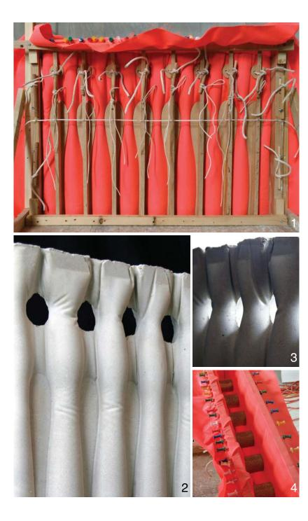
1 Further explorations include a combination of complete perforations and partial-depth impactos, where a space is left between the impactos to form a thin, solid, portion of the wall (2). In this case the impactos may be spaced and restrained from the outside by horizontal beams or buttresses, or by standard wall formties.
